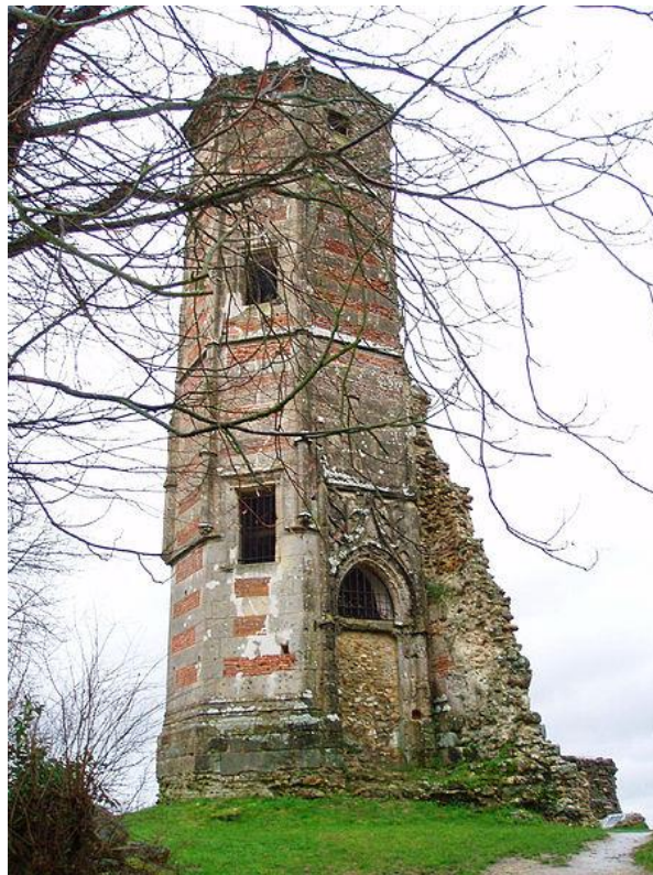
Figure 5.17: Tower of Anne of Brittany (castle at Montfort-l’Amaury) (Photo by User:M-le-mot-dit)
