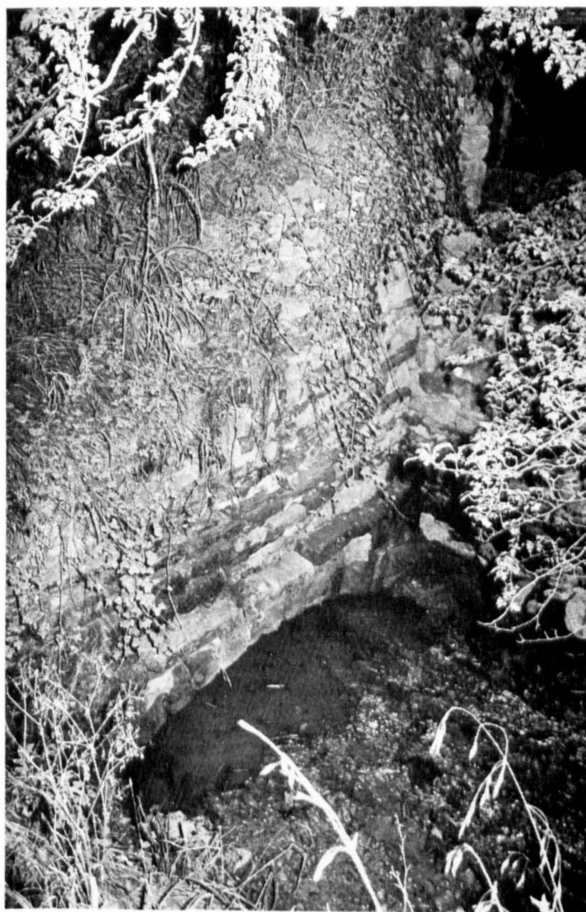
8. The single arch bridge which carries the probable slag mill walls.
