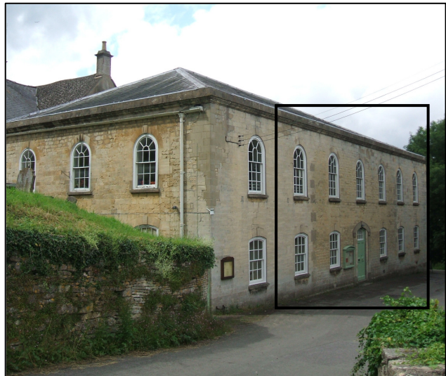
Plate 93: Rodborough Tabernacle, Stroud (2006) – the darker area in the centre is the original 1750 part; the round arched windows on the upper floor were added in 1837.
