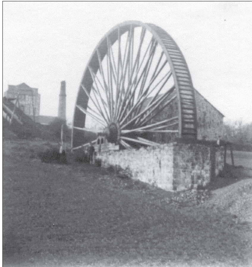
Fig 8.25 Photograph of Arundell Mine, undated but probably from about the 1880s or 90s after abandonment, showing the crusher house. The machinery was powered by a 60ft waterwheel. (see Fig 7.25 for layout). Photographer unknown. (courtesy of Mr & Mrs Heatley)
