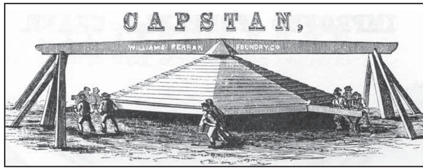
Fig 7.31 A man-powered capstan. From the Illustrated Catalogue of William's Perran Foundry Co. of the 1870s .
