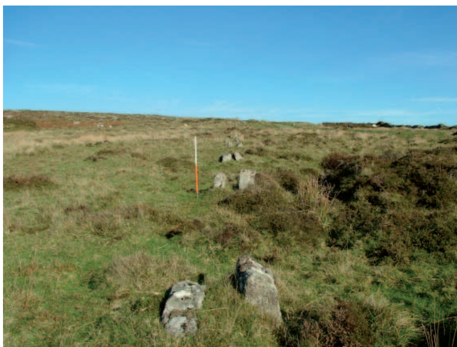
Fig 7.17 Paired granite flatrod supports at Eylsbarrow Mine. Flanged wheels with short stub axles, were supported in grooves in the upper surfaces of the stones.
