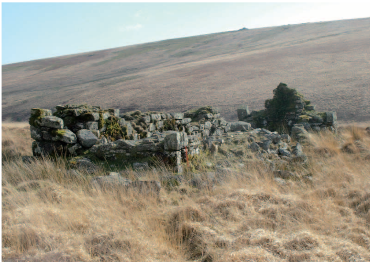
Fig 9.1 A ruined wheelhouse at Huntingdon Mine, which powered pumps via a flatrod system in a shaft 527m to the north.
