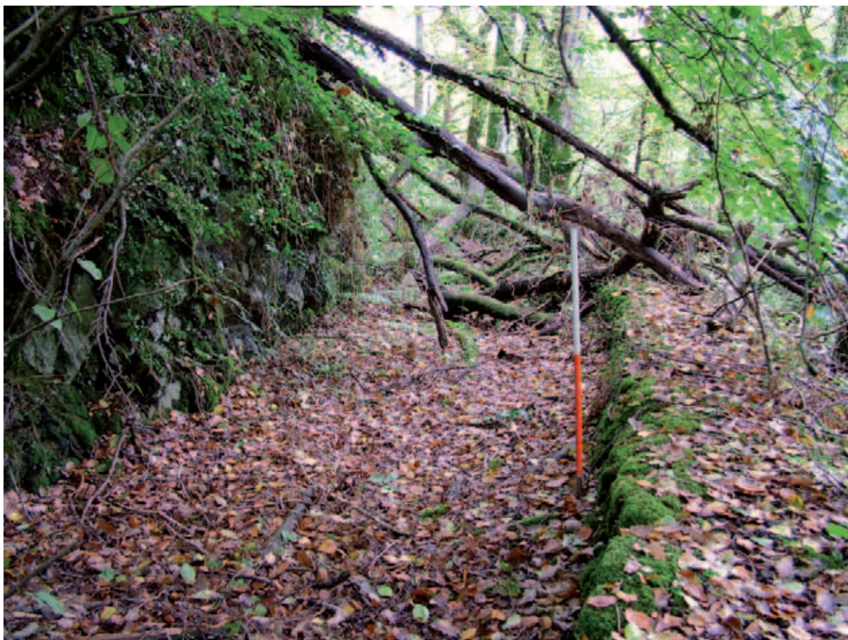
Fig 9.3 A disused section of rock cut leat which diverted water from the River Dart to Queen of the Dart copper mine.
