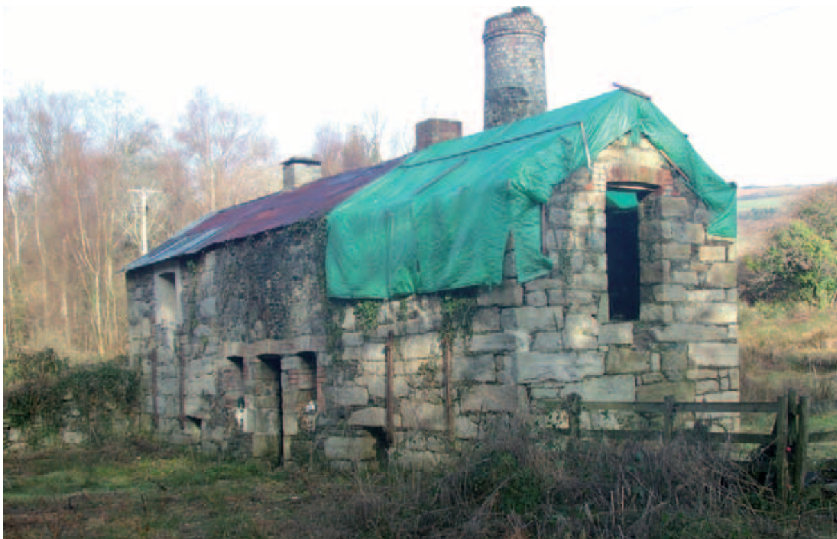
Fig 8.21 The burning house at Atlas in 2009. Although the upper story of the burning chambers is covered and roofed, the layout of this late 19th century examples differs little from that pictured in Angerstein's drawing of 1753 (Fig 8.18). However, as with most later examples, a chimney is attached at the rear of the building.
