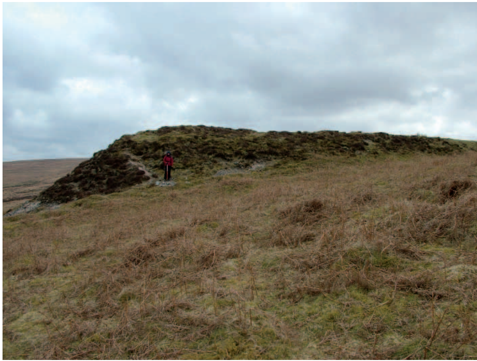
Fig 7.36 A large finger dump of mine waste emanating from Lowe's Shaft at Hexworthy Mine. The flat upper surface would have accommodated a tramway.
