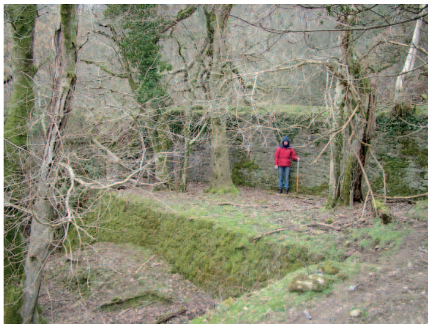
Fig 8.11 The substantial retaining wall and ore-dumping area at Crownley Parks dressing floors, part of Haytor Consols.
