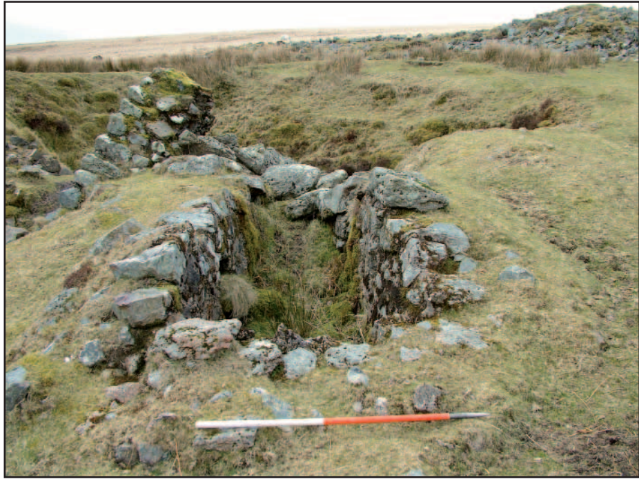
Fig 7.21 A masonry lined bob pit at the head of Lowe's Shaft, Hexworthy Mine. The conical dip in the ground just beyond the pit is the head of the shaft.
