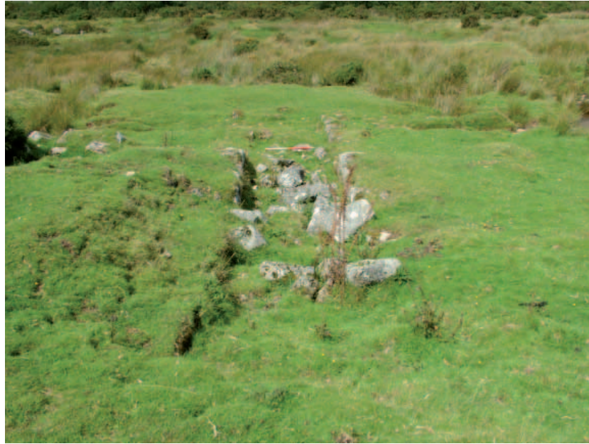
Fig 8.7 A sunken stamps wheelpit at Gobbett mine which has been part demolished and backfilled.
