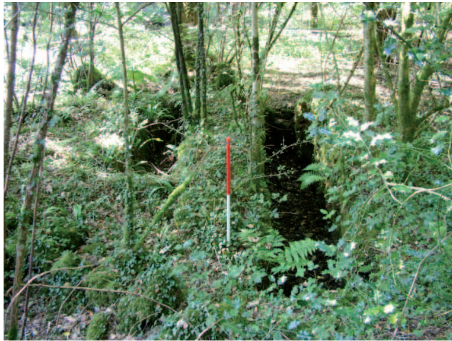
Fig 7.27 Overgrown wheelpit for a waterwheel to power a whim, with the characteristic drum pit on the left hand side. Little Gem Mine.
