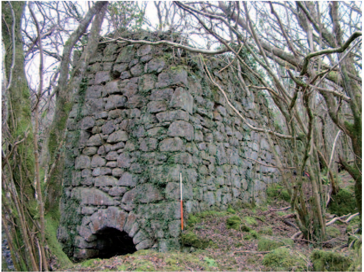
Fig 9.2 A partly ruined wheelhouse at Great Wheal Eleanor which provided power to a flatrod system as well as supplementing a steam engine to power a stamping mill. The moss-covered revetment of the dressing floor is visible on the right.
