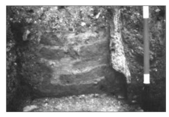
Fig 4. Excavations at Blue Boar lane 1958. Section through north wall of courtyard showing detail of clay brick structure with plaster facing, right (*Wacher site archive*, *University of Leicester*).
