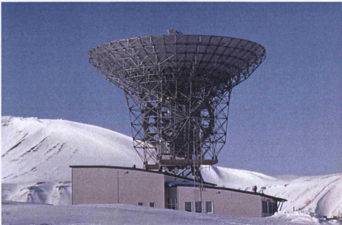
Figure 3.13. ( Top panel ) The EISCAT site at Ramfjordmoen near Tromsø, Norway. The VHF antenna is on the left and the 32 m UHF antenna is on the right, adjacent to the buildings that contain the transmitters and control equipment. ( Lower panel ) The buildings and 32 m steerable antenna of the ESR at Longyearbyen, Svalbard (Photographs courtesy of EISCAT).
