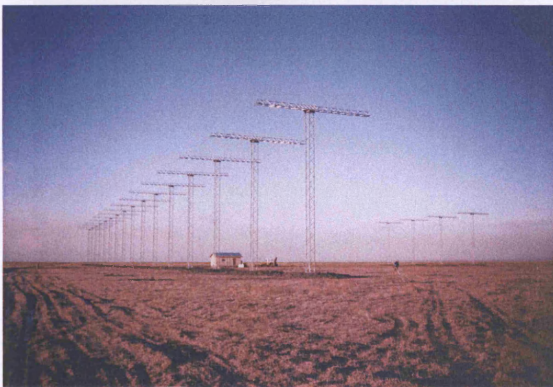
Figure 3.5. The CUTLASS Finland (top) and Iceland (bottom) radars. The four antennas of the interferometer array and equipment building that contains the transmitters and control computers are clearly visible at the Iceland site whilst they are hidden by trees at the Finland site (Photographs provided by E. Chris Thomas, University of Leicester).
