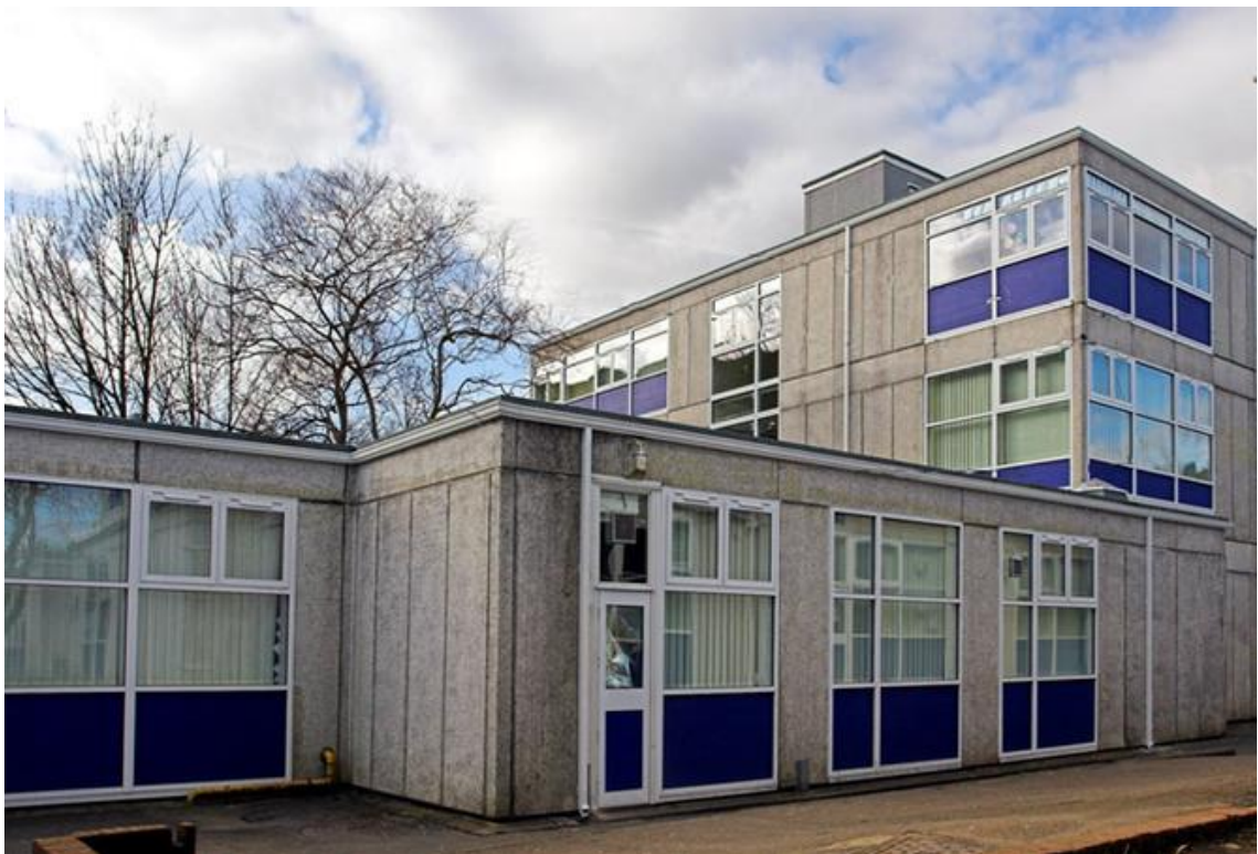
Figure 2.3 A CLASP modular school build
