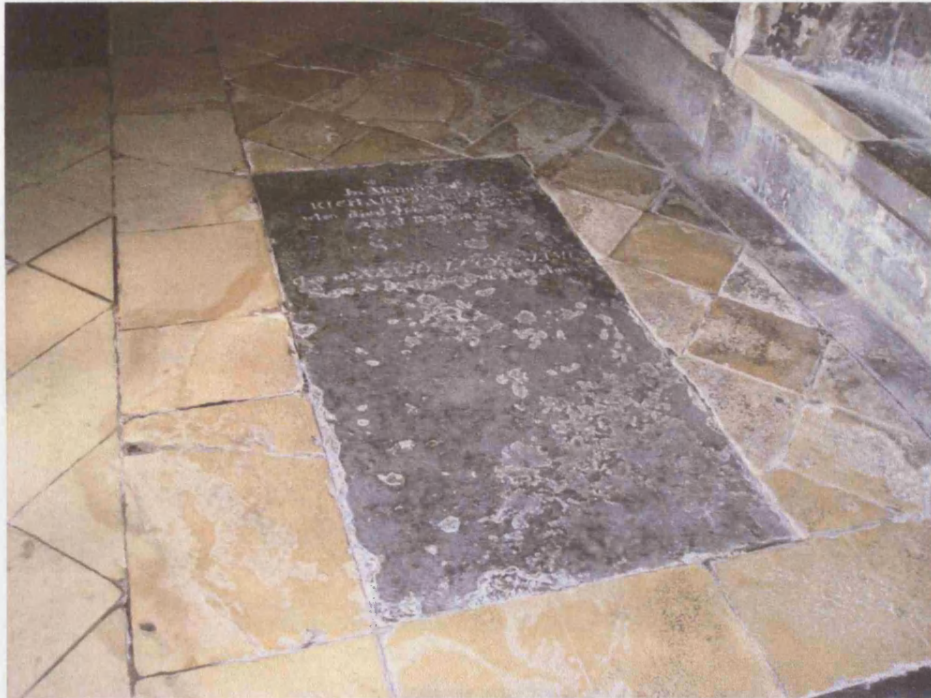
Figure 7.20: A badly degraded ledger in the Cloisters at Gloucester Cathedral.
