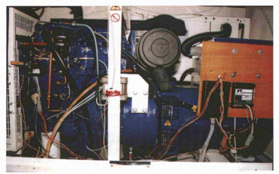
Picture 4. Diesel generator set, left hand side, showing air filter pipe-work, oil filter, controller, actuator and fuel pump.
