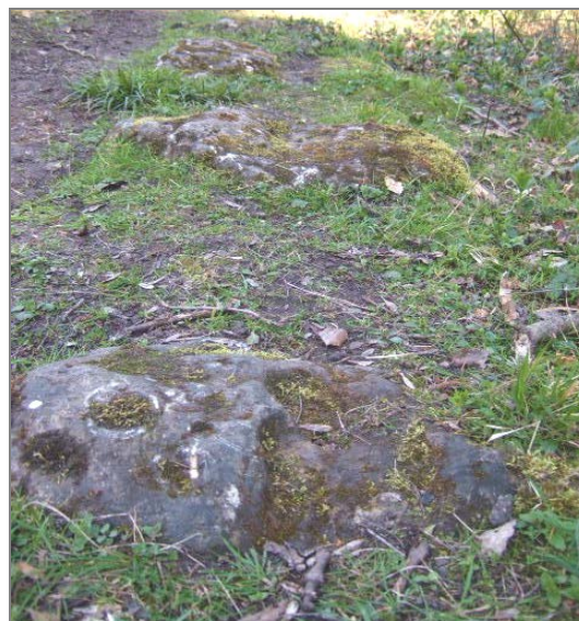
Figures 76 and 77: The remains of the embankment and stone sleepers upon which the tramways ran.
