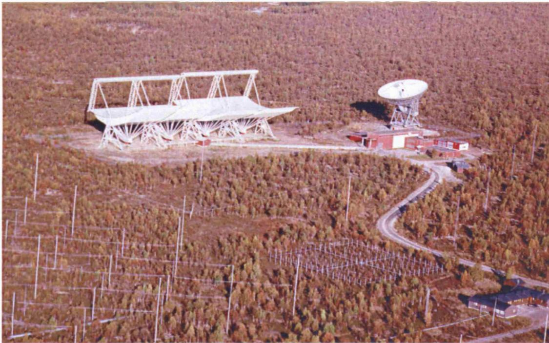
Figure 4.12: The EISCAT site at Tromsø. The UHF and VHF EISCAT incoherent scatter radars are visible in the upper part of the diagram. The lower left of the picture shows a part of the heater array. This is controlled from the heater building visible in the lower right of the picture.
