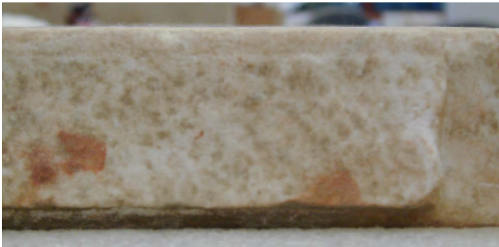
Figure 29: Base of Robert Hill's tombstone showing remnants of tenon and tool marks made during straightening of base (photo by author).
