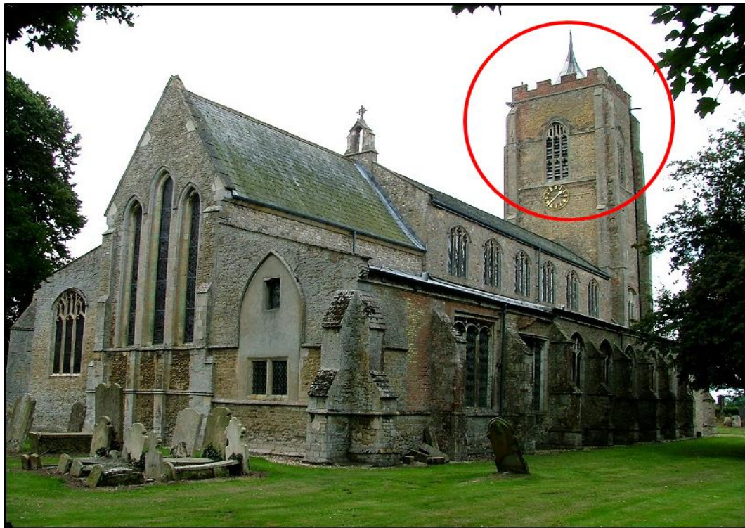
Figure 4.8 – Emneth Church showing late medieval ‘Dutch’ brickwork in the tower (author’s photograph).
