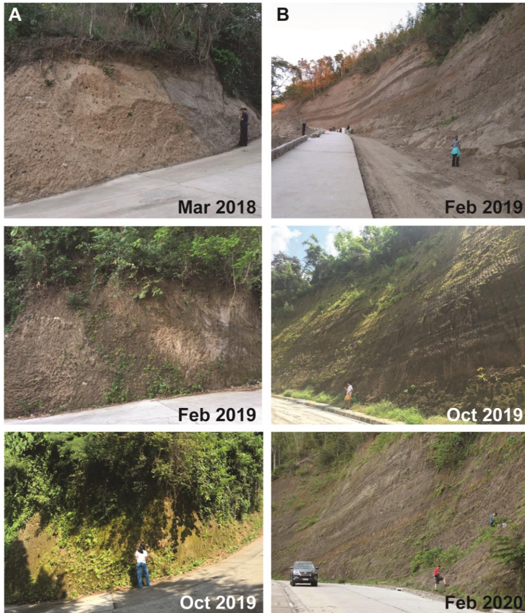
Fig. 1.6: (A) An exposure along Tagaytay Ridge freshly exposed in March 2018, showing a dark weathered surface in February 2019 and covered in thick vegetation during the rainy season in October 2019. (B) An exposure along the southern shore of Lake Taal freshly exposed in February 2019, covered in vegetation and a weathered surface during the rainy season in October 2019, and in the dry season in February 2020.
