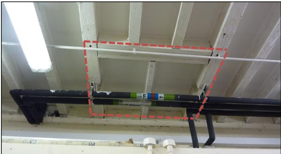
Figure 6.24. Cut-out (now blocked) for a hoist in the ceiling of the storeroom at the GSK, Newcastle-upon-Tyne to the kitchen above.
