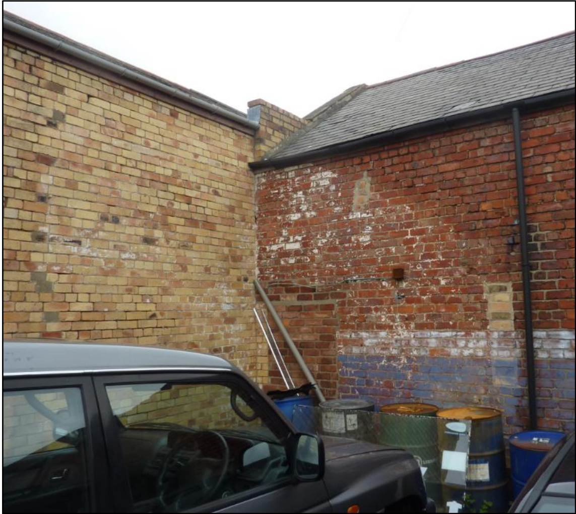
Figure 8.19. The site of the pot house, Pegswood Co-operative Society; the blocked door to the slaughterhouse and repairs to the wall are visible with traces of whitewash and less weathered brick.
