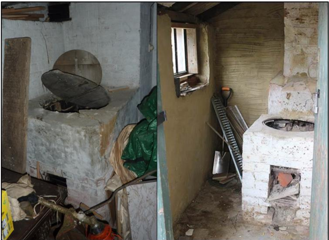
Figure 6.21. Left stove at the Manor with a capacity of about 120 quarts and the two wooden covers. Right stove at Manor Farm with a capacity of about 50 quarts.
