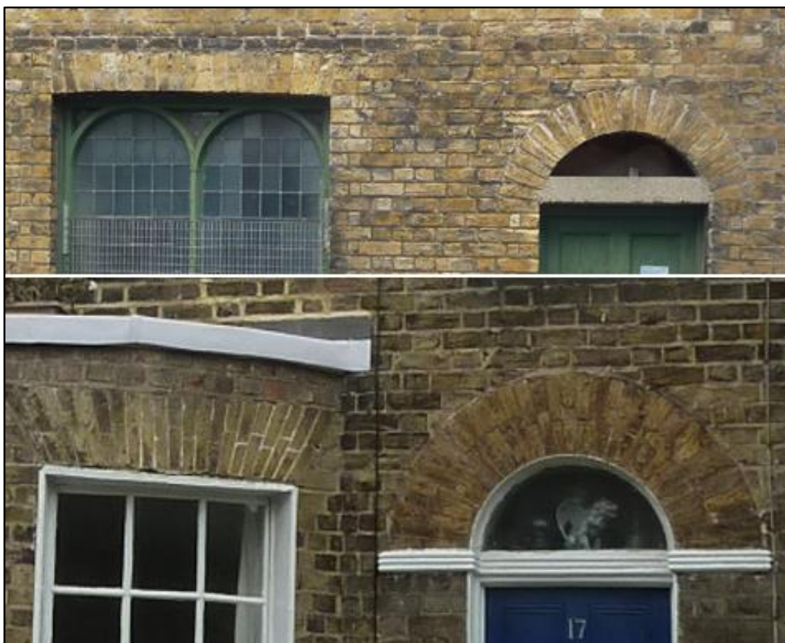
Figure 7.19. Above detail from the façade of the soup kitchen, below a contemporary nearby house with a more finely formed window lintel and fanlight.
