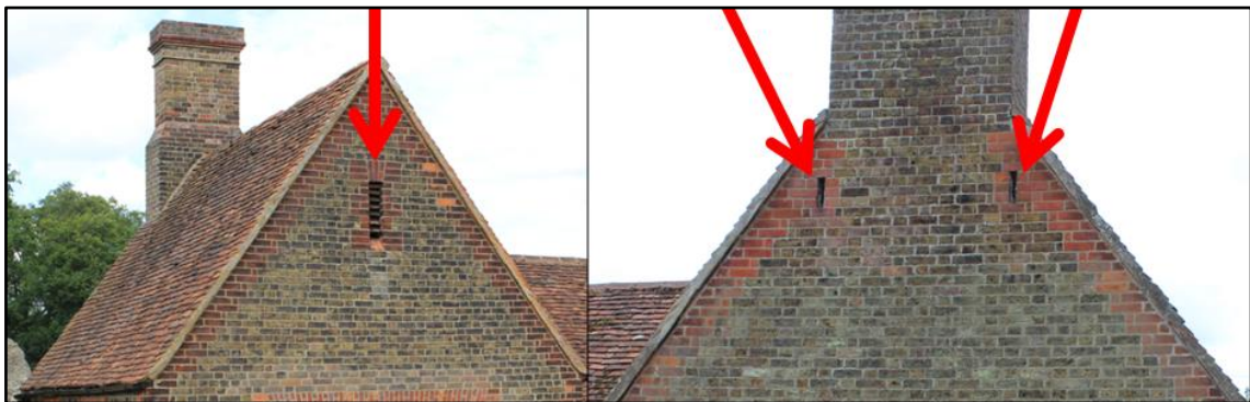
Figure 6.29. The Soup House, Berkhamsted, Hertfordshire: ventilation slots in end gables, left front, right rear.
